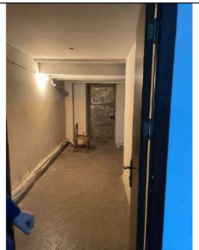
Additional entrance to the basement
